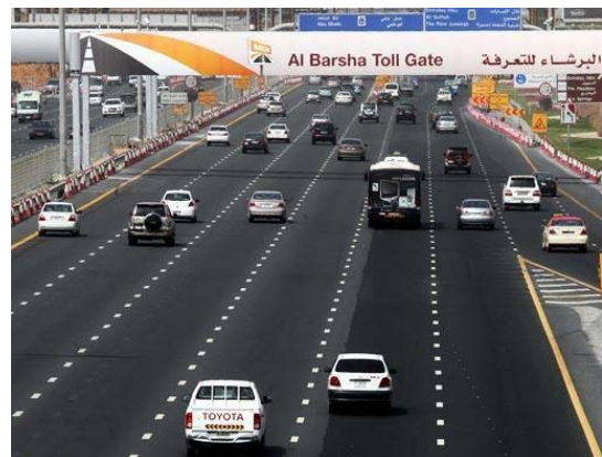
Figure 2. Sample Salik toll gate [12].
